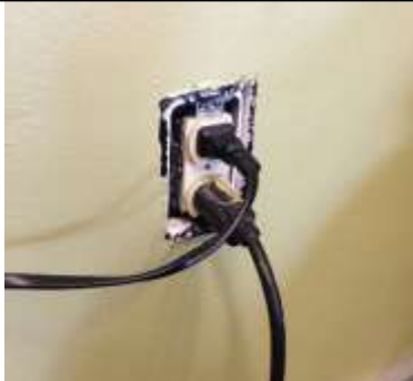
MISSING ELECTRICAL PLATE
