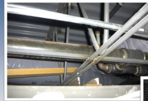
Open-web steel bar joist w/ metal roof decking
