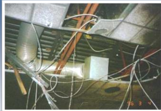
These obstructions and false ceiling grids can fall and become entanglement hazards for fire attack crews
