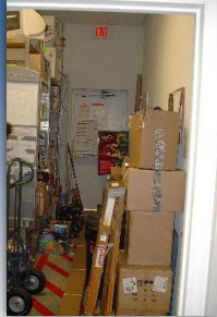
“Temporarily” blocked aisles can limit avenues of ingress and egress
