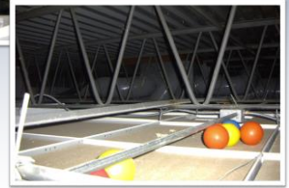
Open-web steel bar joist w/ metal roof decking
