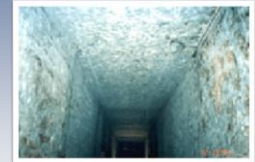
Cleared ductwork
